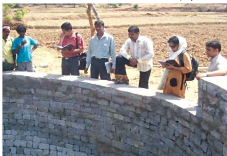
One of the five wells constructed in the project area
